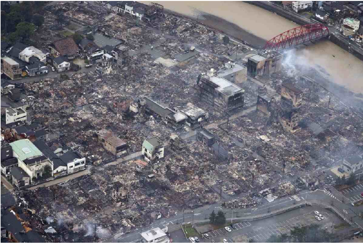
Figure 1: Aerial footage of Wajima in the aftermath of the earthquake [1]
